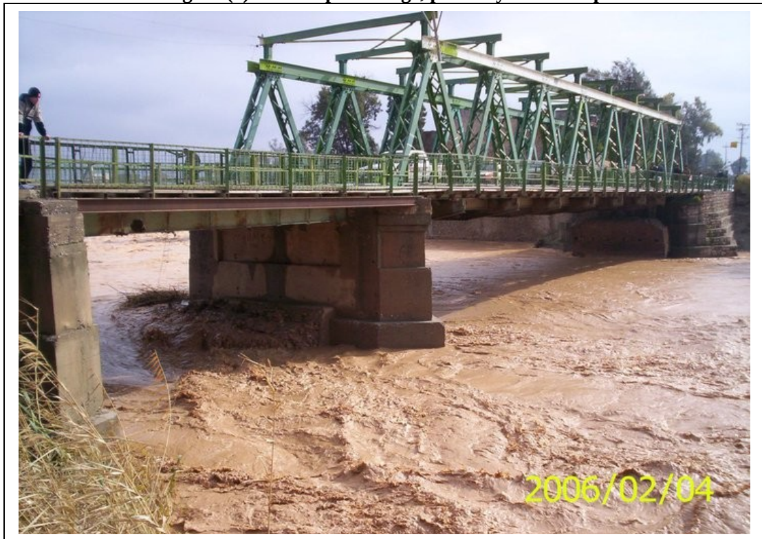
Figure (4) Altunköprü Bridge, photo by Ali Kassap
