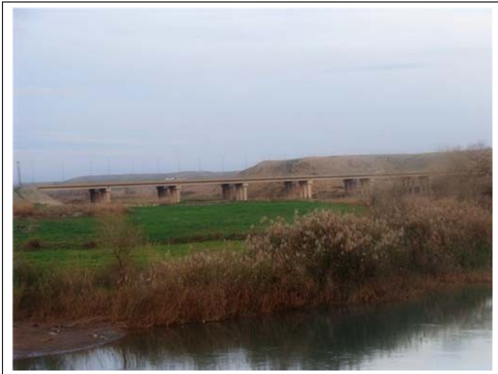
Figure (14) scenery from Altunköprü
