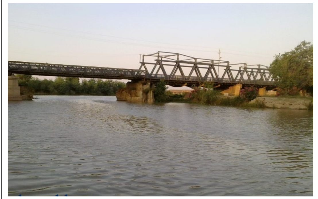
Figure (3) Altunköprü Bridge, photo by Ali Kassap
