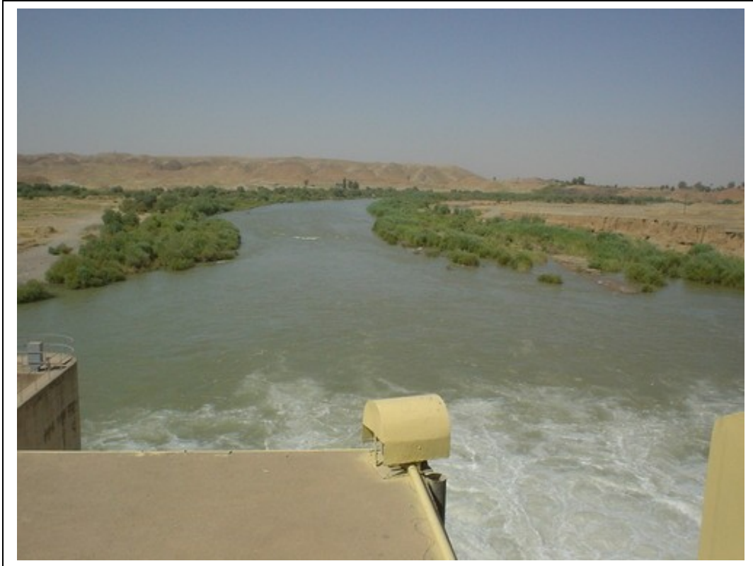
Figure (12) Dibilis Dam photo by panoramio.com
