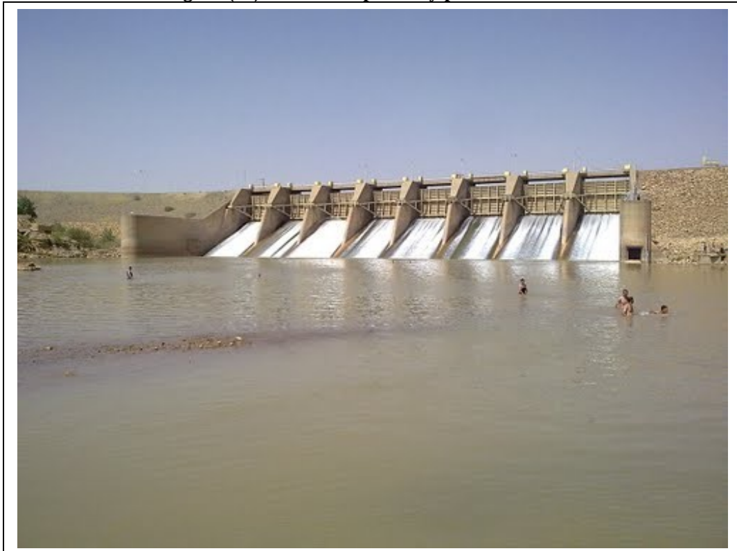
Figure (13) Dibilis Dam photo by panoramio.com. The dam is located directly north of the district of Dibilis (Numera Sekiz) in Kirkuk. The main-purpose of the Dibilis Dam is to divert water from the little Zab River into the Kirkuk Irrigation project.
